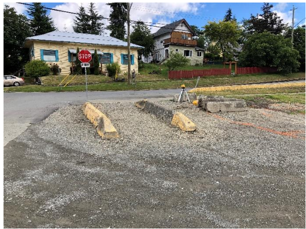
Site Location – looking north
