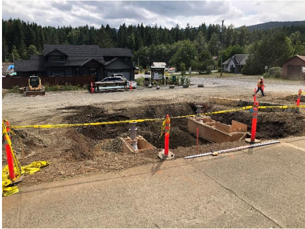
Site Location - looking south
