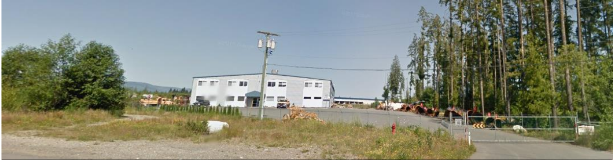
Photo 1: View from Royston Road - existing facility & fencing
