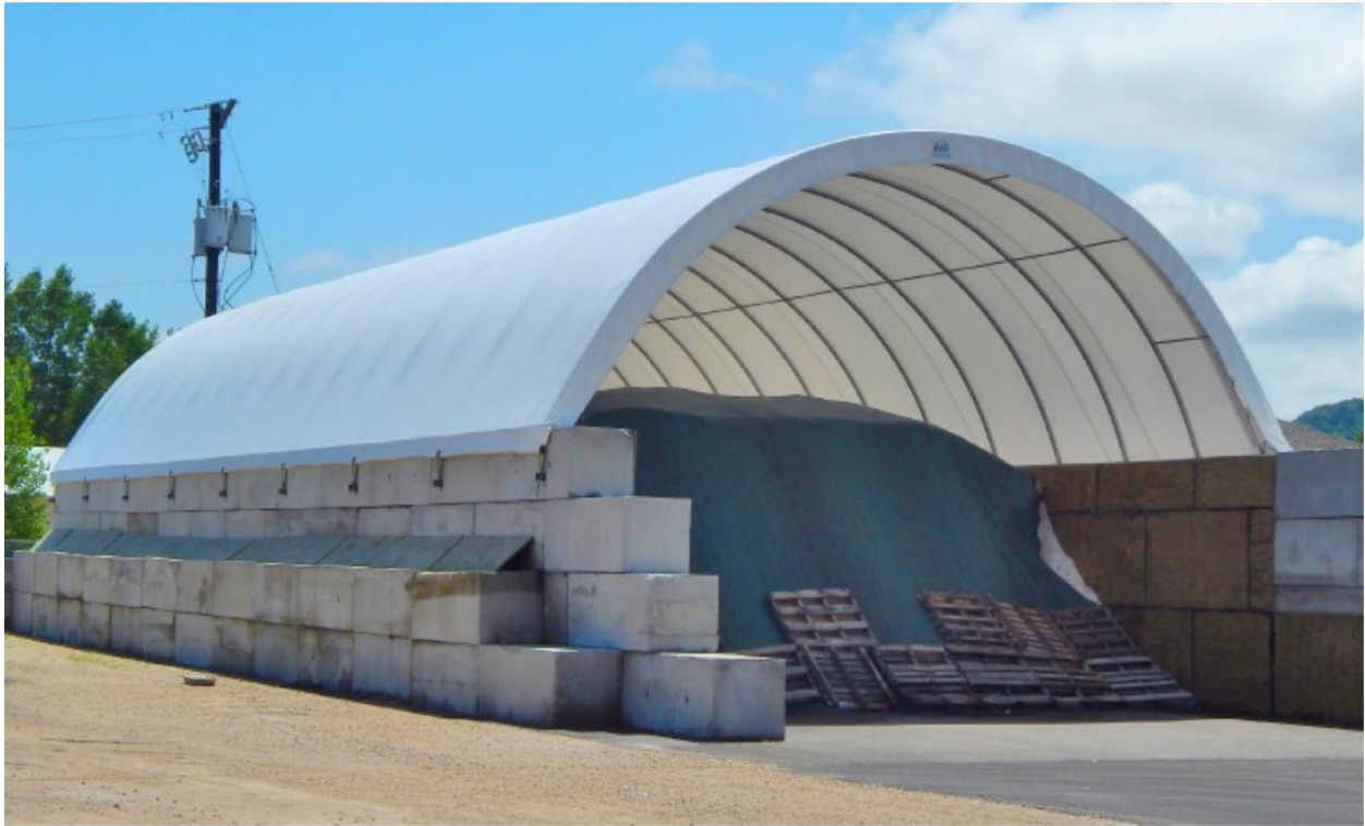
Photo 3: Image of a similar storage shed
