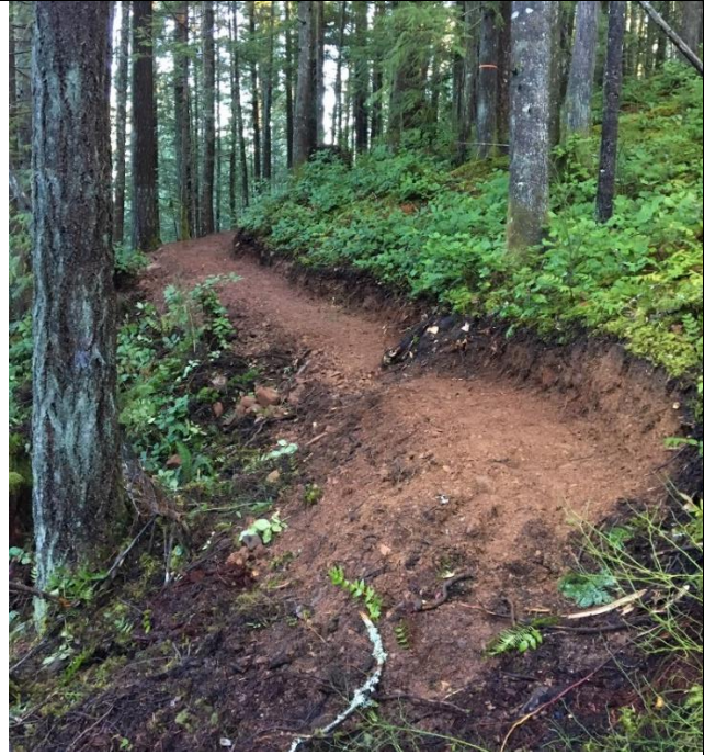
Bench cut trail construction on Two and a Juice re-route project (Cumberland Community Forest.)
