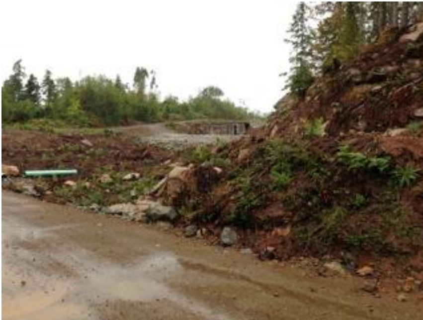
12. Approach into canyon from the south with Fan house in center
