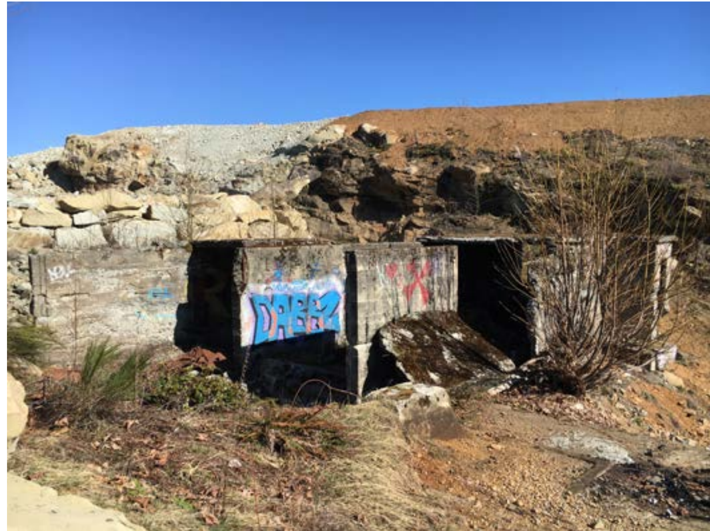
VIEW FROM EXISTING ROAD - LOOKING NORTHWEST
