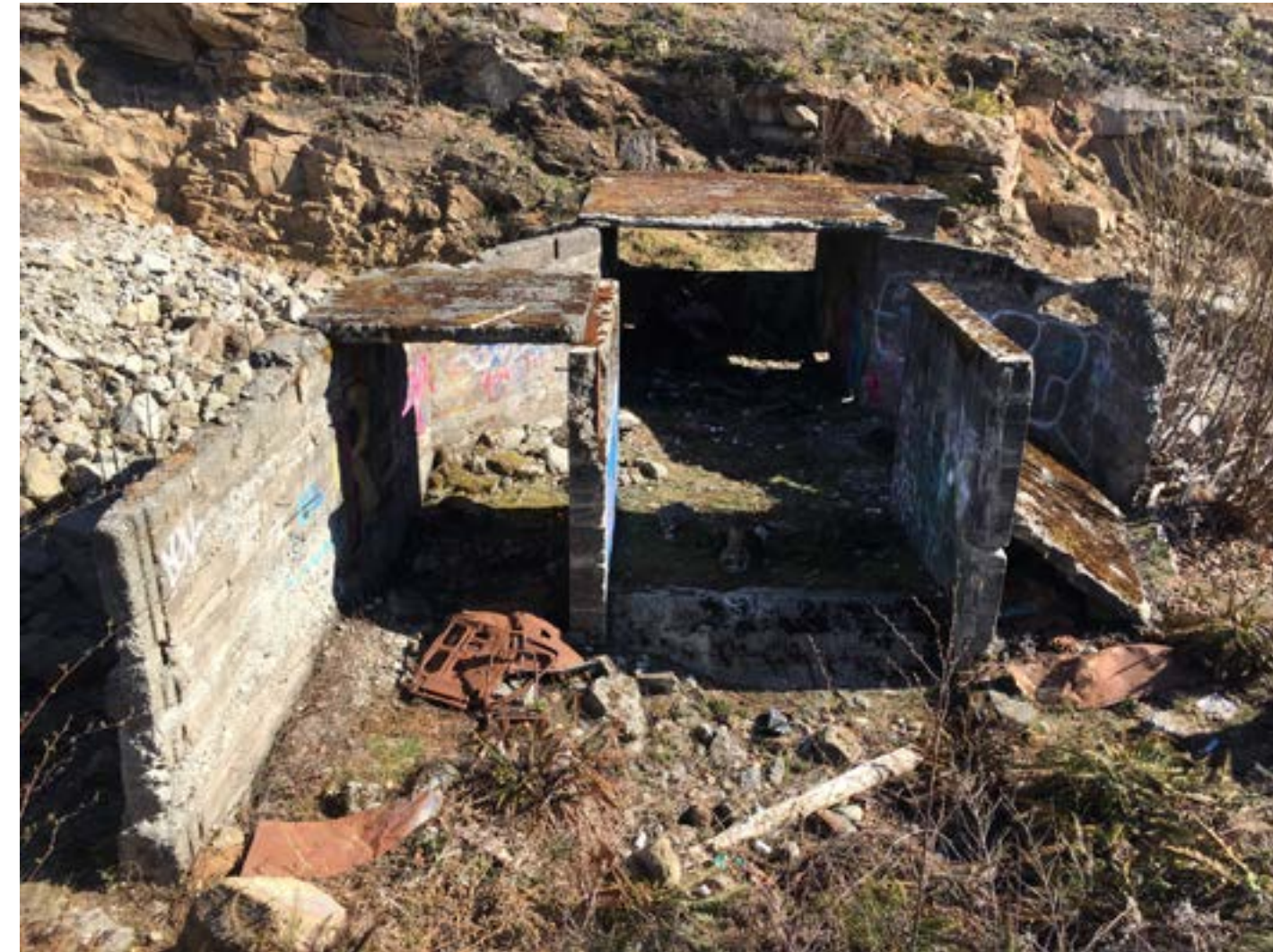
VIEW FROM ROAD - LOOKING WEST
