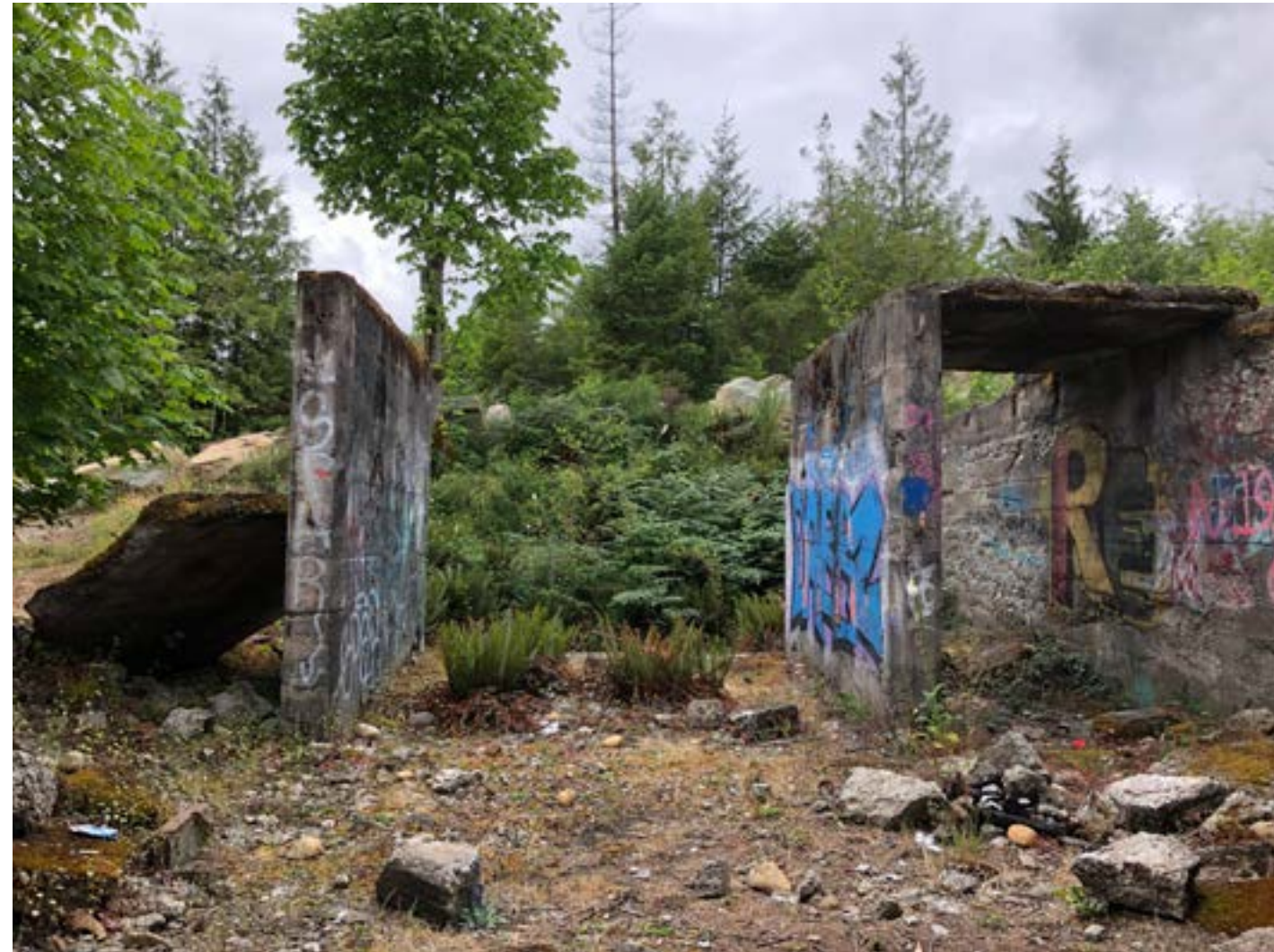
MAIN AIR SHAFTS - LOOKING WEST
