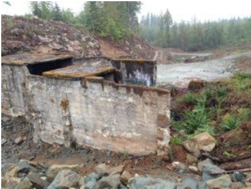
3. From north looking down canyon with north exterior wall
