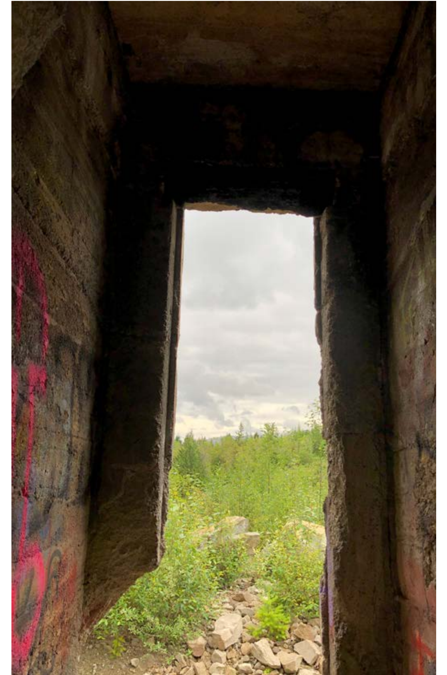
LOOKING SOUTH THROUGH ACCESS DOOR
