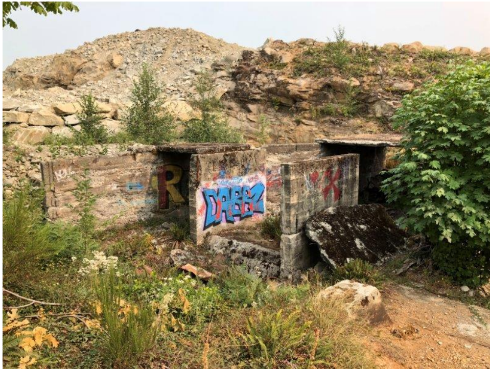
Photo 2 General View of Fan House Building
