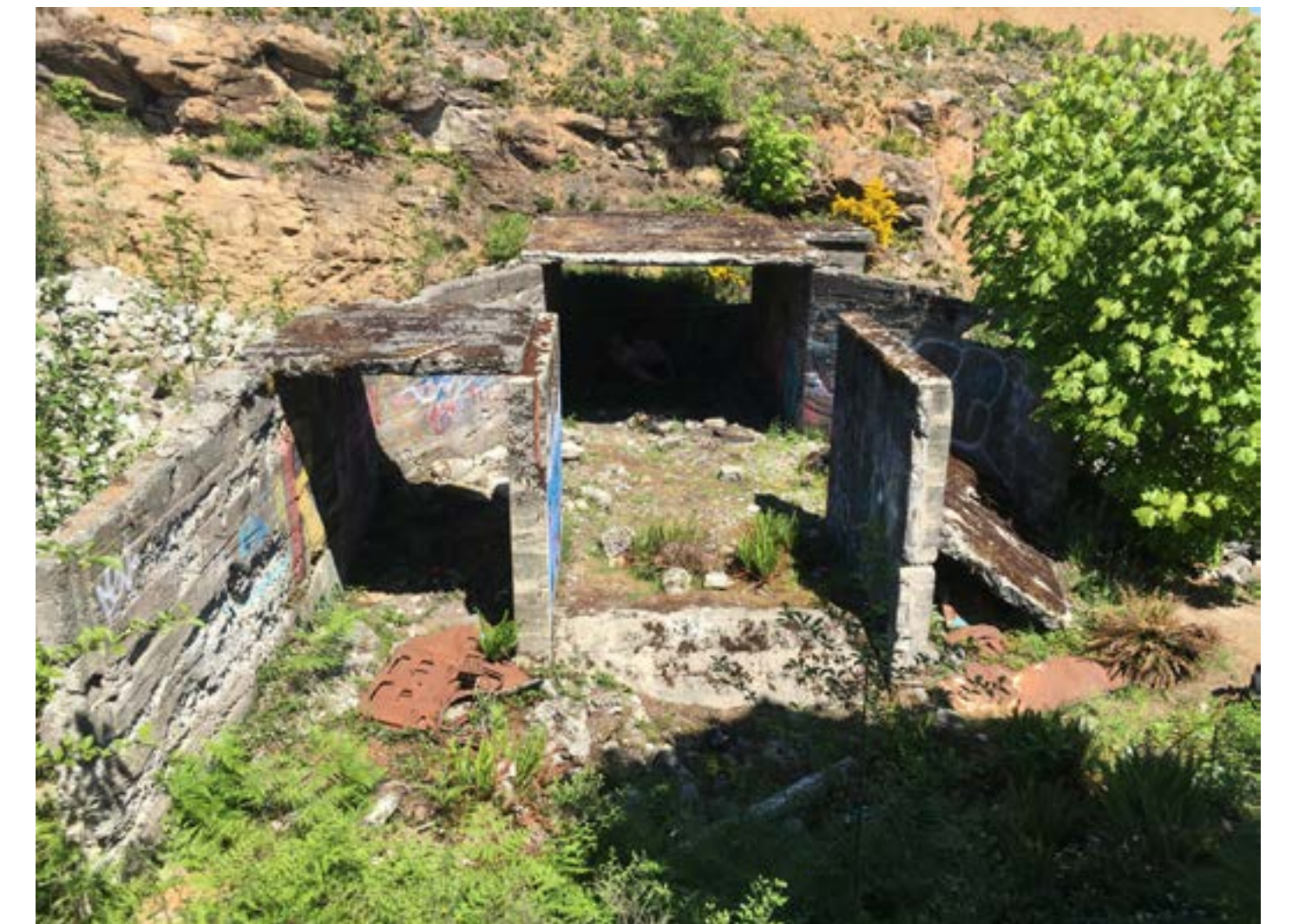
VIEW FROM ROAD - LOOKING WEST
