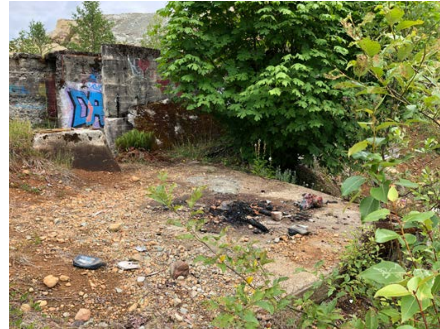
BUILDING SLAB WITH CONCRETE PIER
