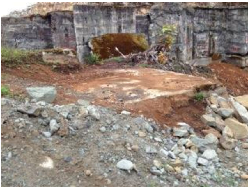
10. Concrete slab to south of main structure
