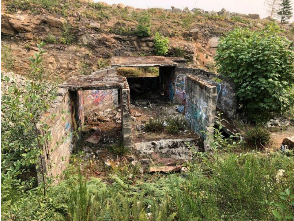
Photo 1 General View of Fan House Building
