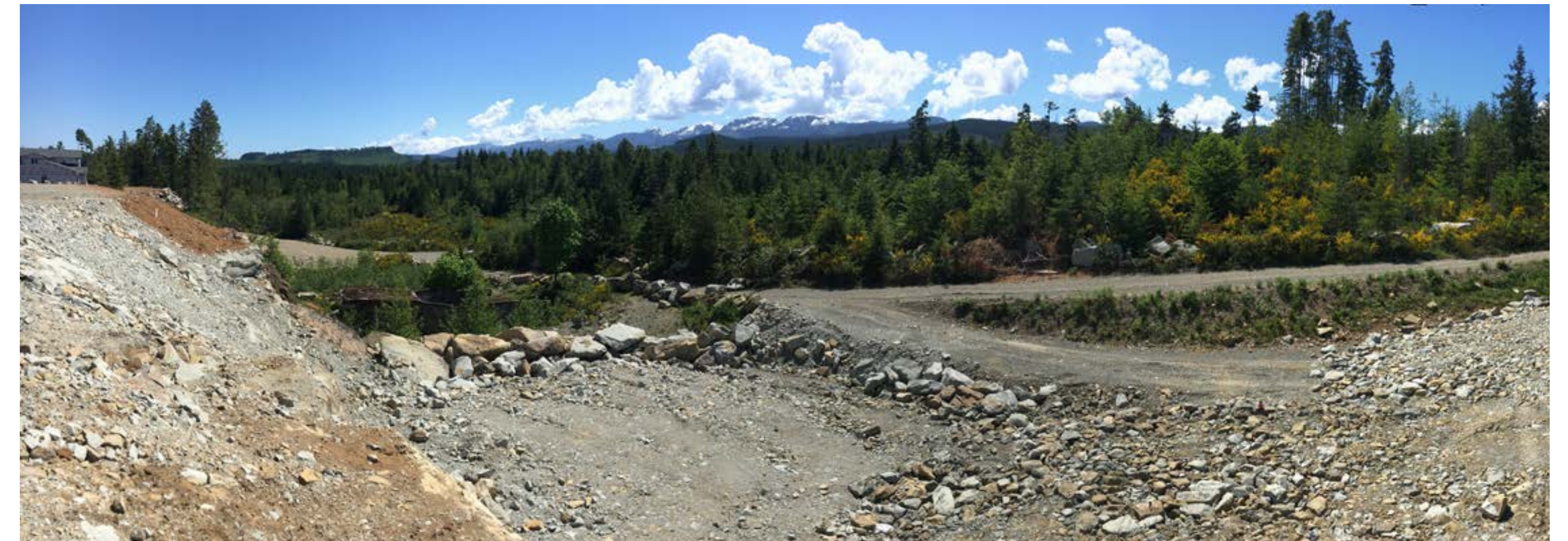
VIEW EXISTING UPPER LOTS - LOOKING SOUTH
