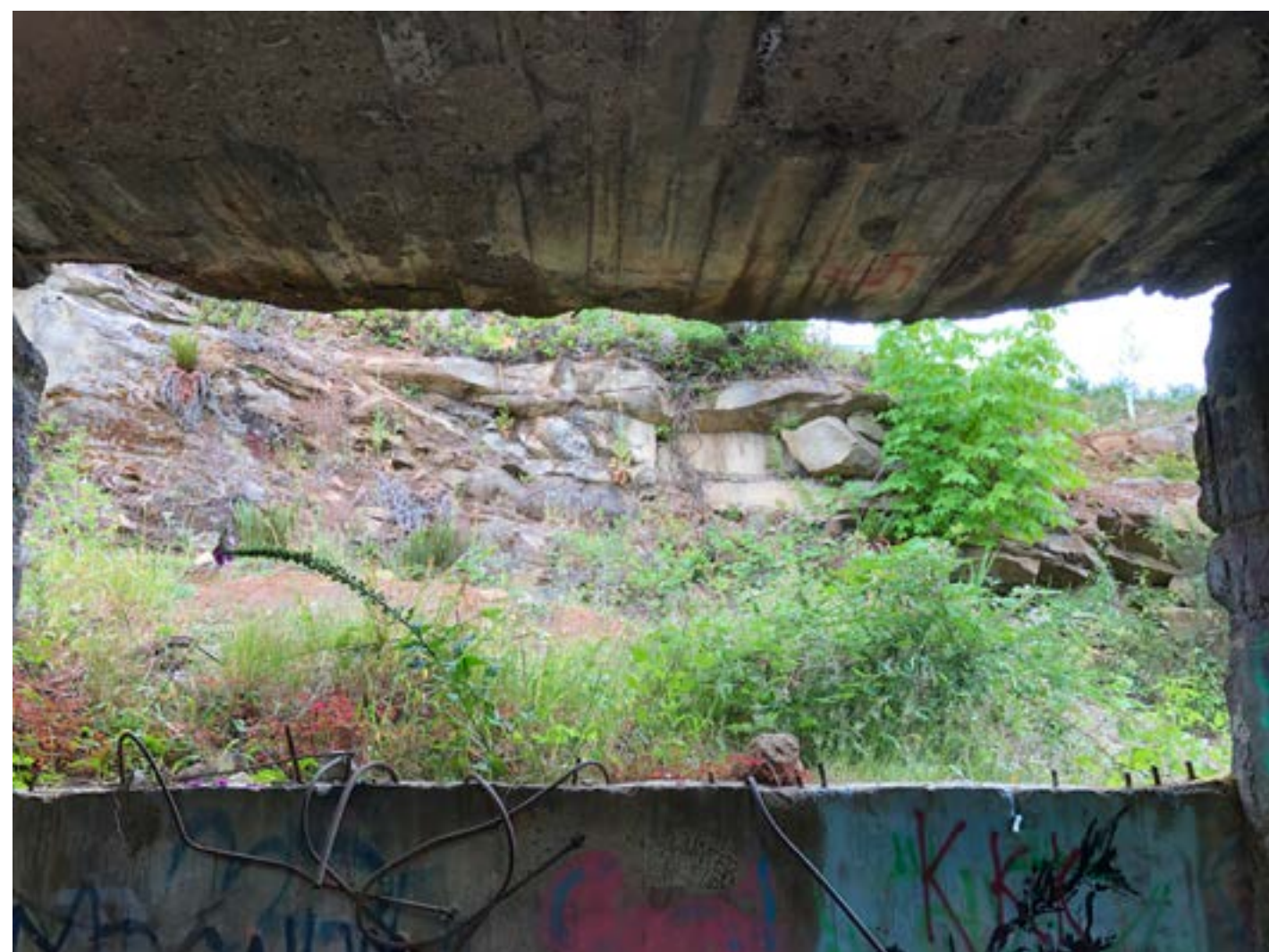
LOOKING EAST THROUGH VENT SHAFT
