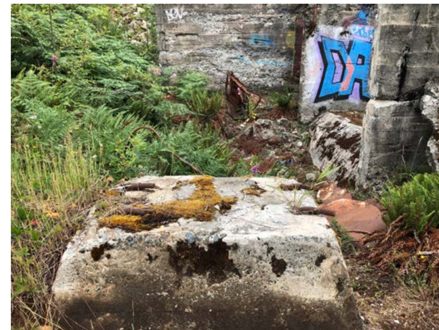
CONCRETE PIER AND THREADED BOLTS
