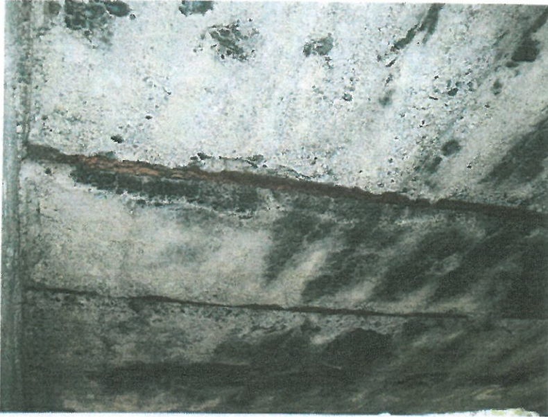
Photo 1 – Channel Reinforcing in Roof Slab
