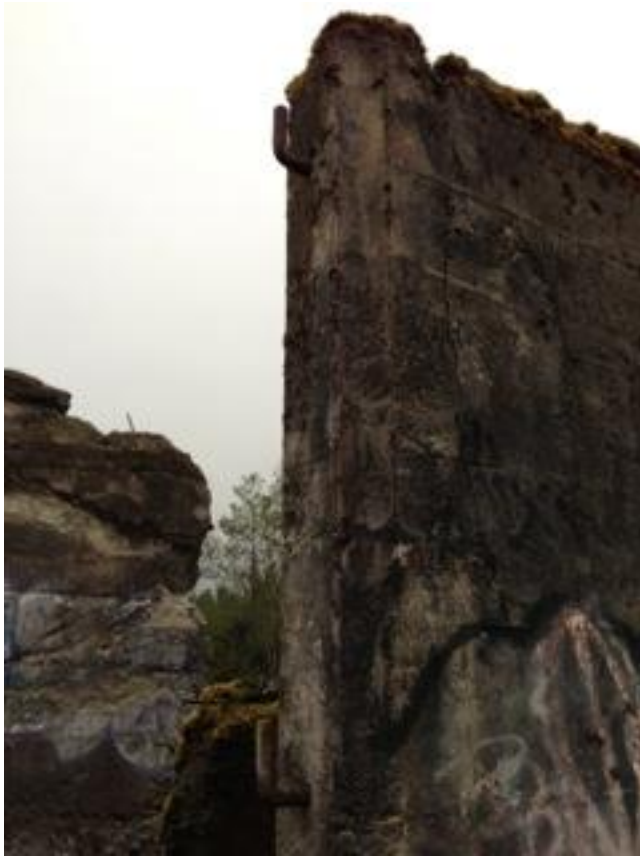
9. Fin wall showing two metal hinges
