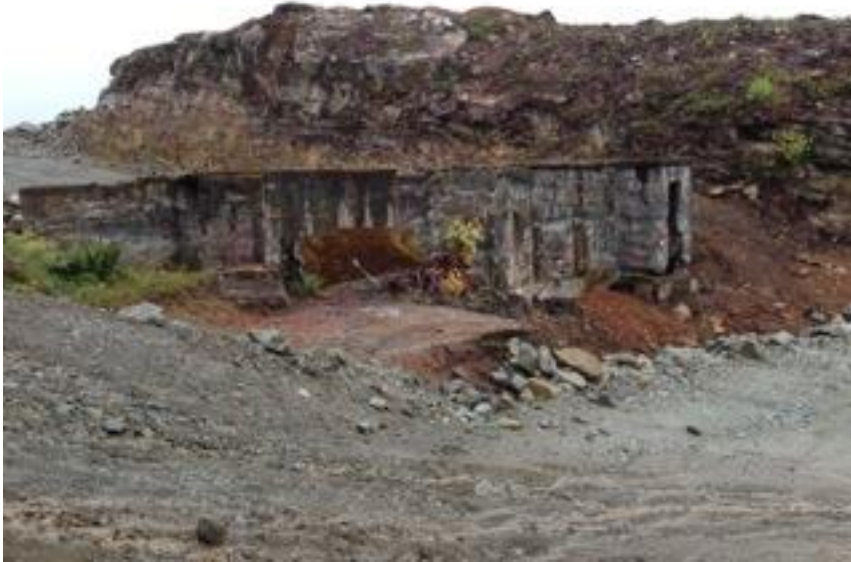
16. From the west all vegetation removed
