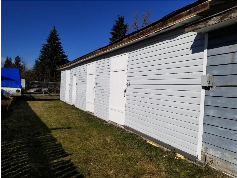
North side of Mini-Storage Building, recently repainted
