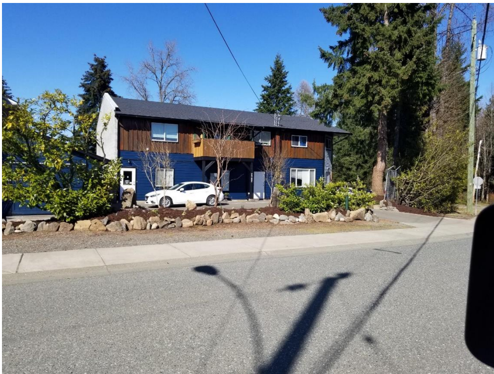
Existing 4-plex from Ulverston Avenue
