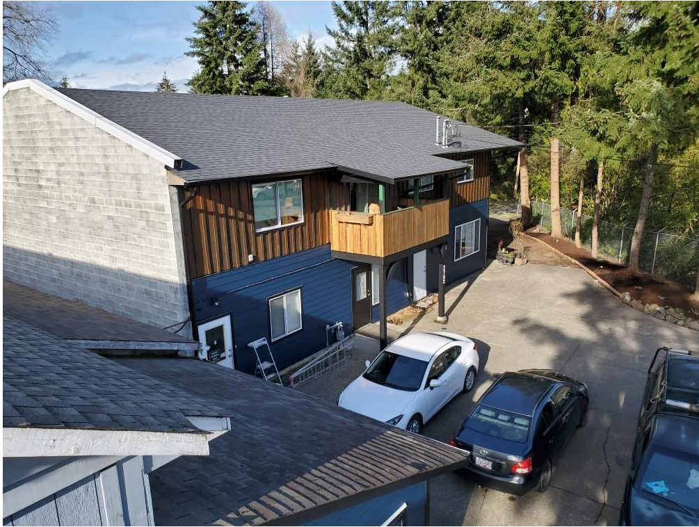
View of existing 4-plex from top of mini-storage building
