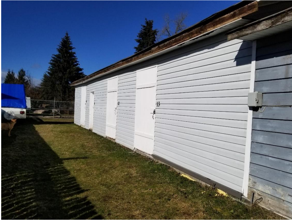
North side of Mini-Storage Building, recently repainted
