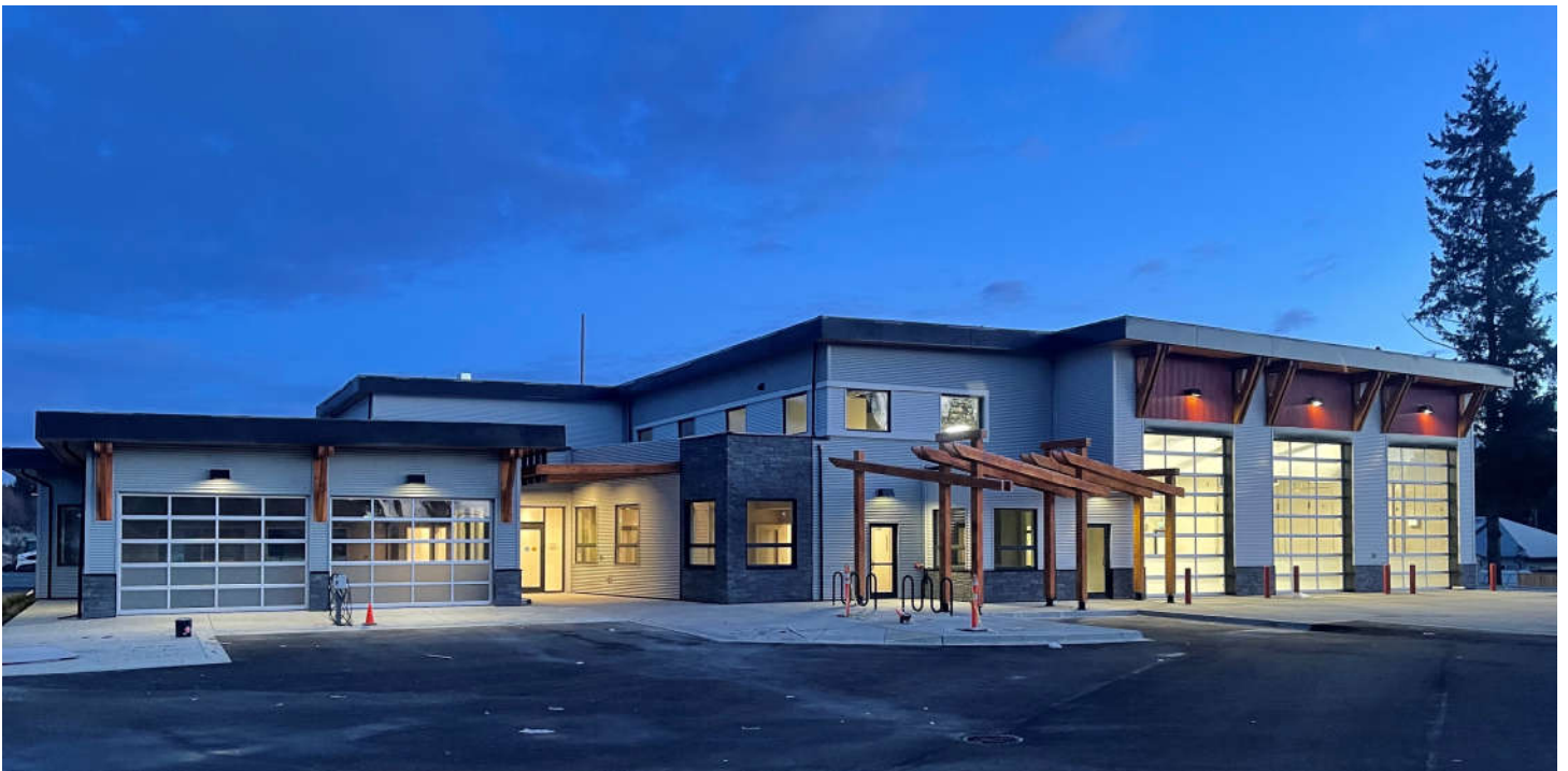
The new fire hall nearing completion.
