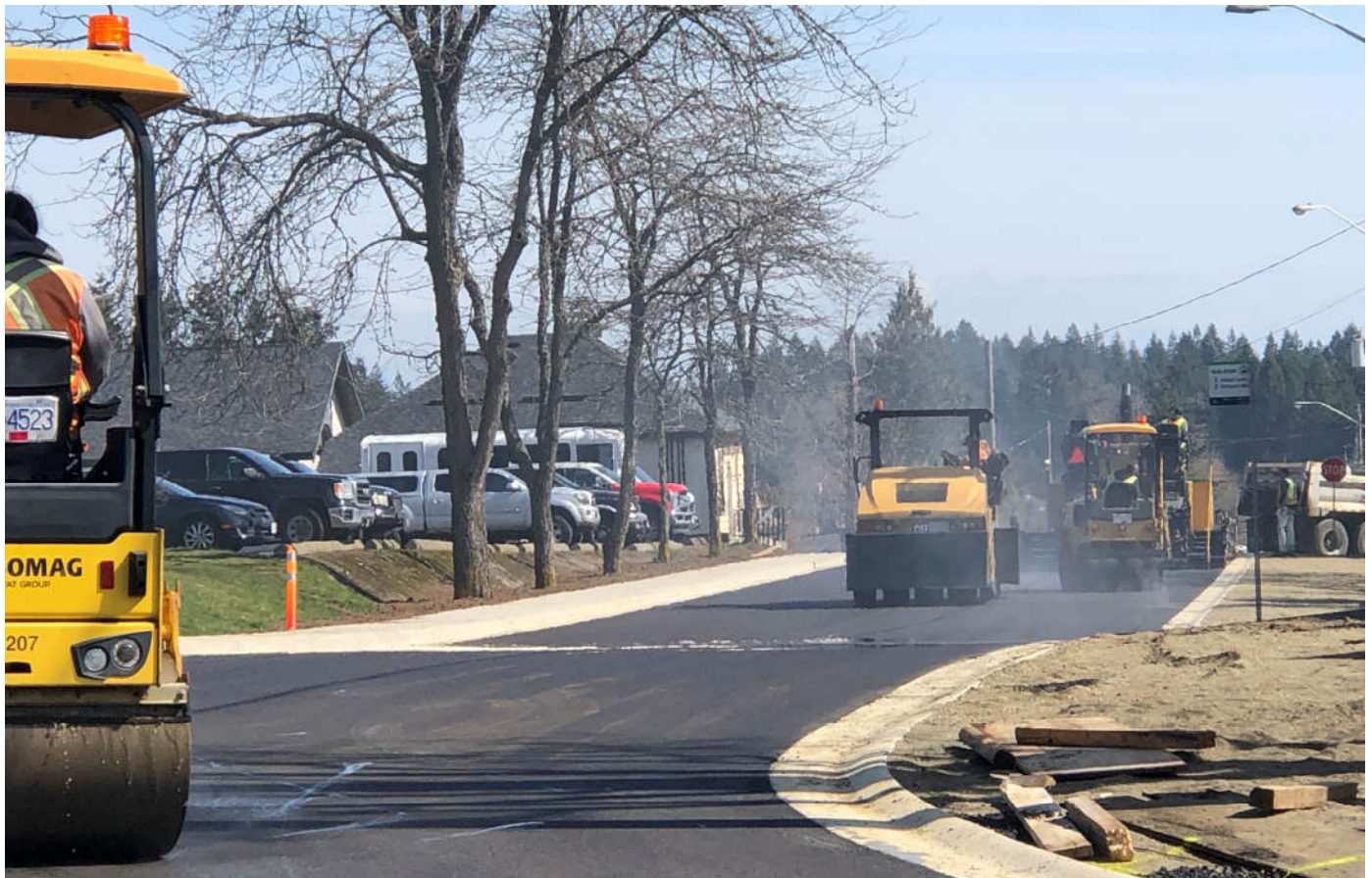
Construction in final stages on Windermere Avenue
