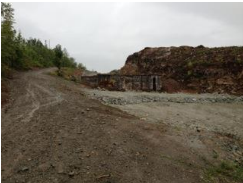
14. Canyon and Fan house from the south
