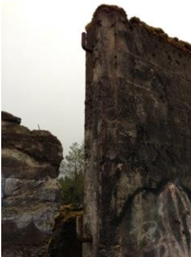
9. Fin wall showing two metal hinges
