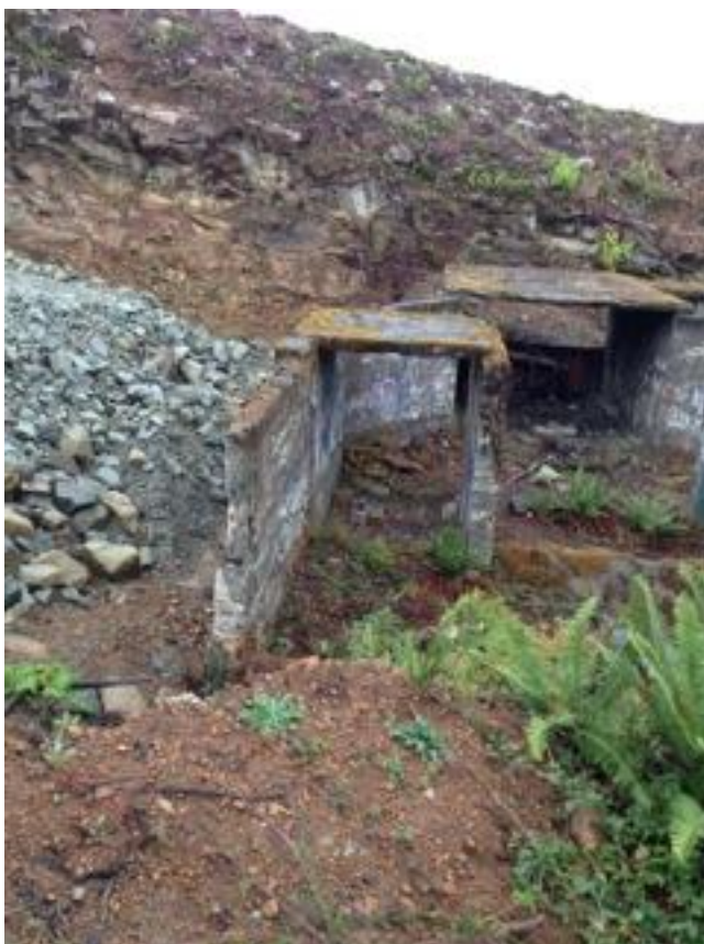
15. Looking across canyon to the east, note fill to left
