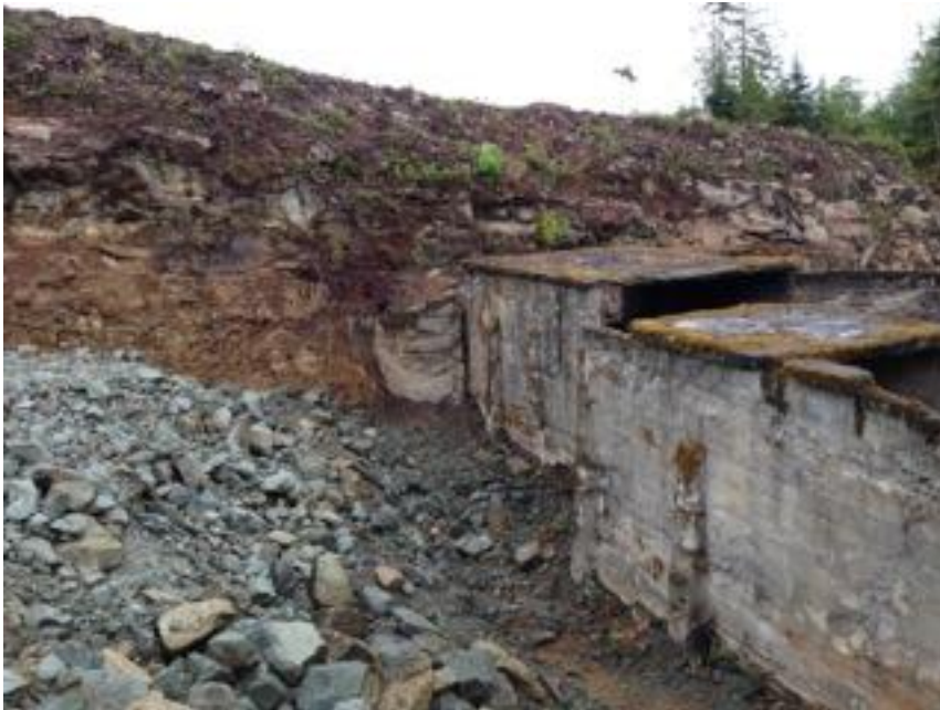
20. Placement of blasted rock fill to north side of Fan house
