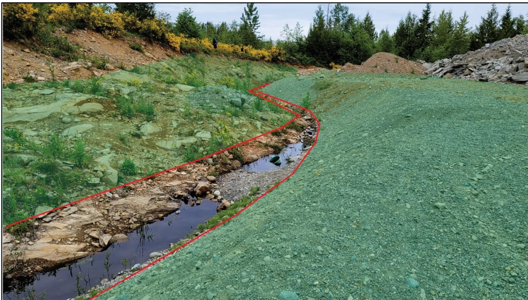
Figure 3: View to northeast showing approximate high water mark in red and restoration areas shaded green. Invasive plants should be removed, topsoil added and native vegetation planted.
