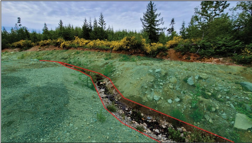
Figure 4: View to southwest showing approximate high water mark in red and restoration areas shaded green. Invasive plants should be removed, topsoil added and native vegetation planted.
