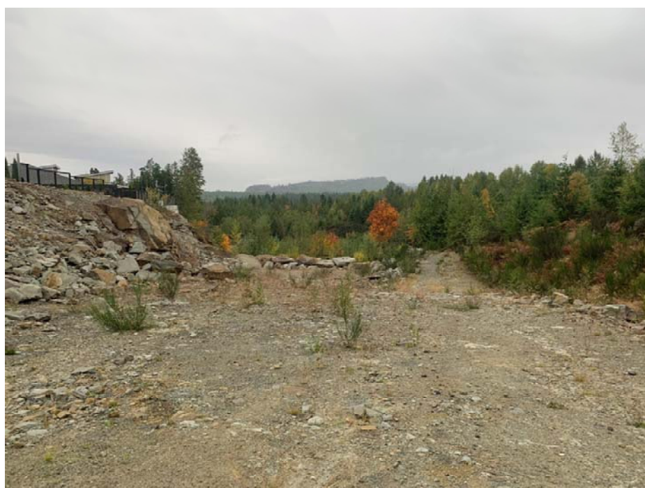
Future Road near Old Fan House
