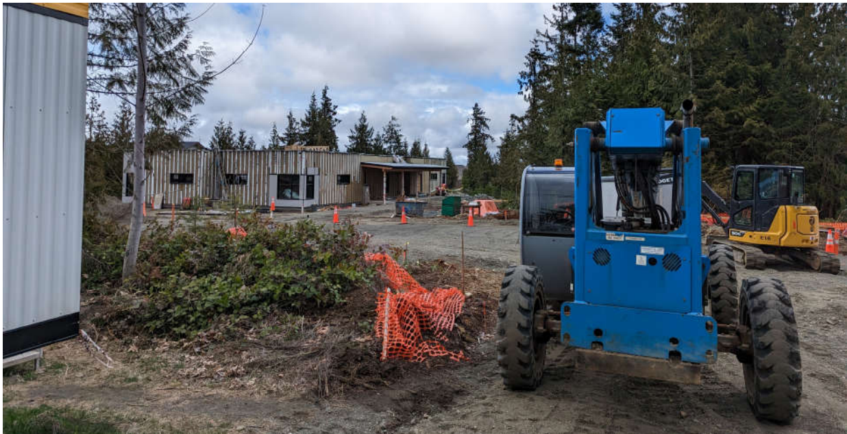
Cumberland Child Care Centre under construction
