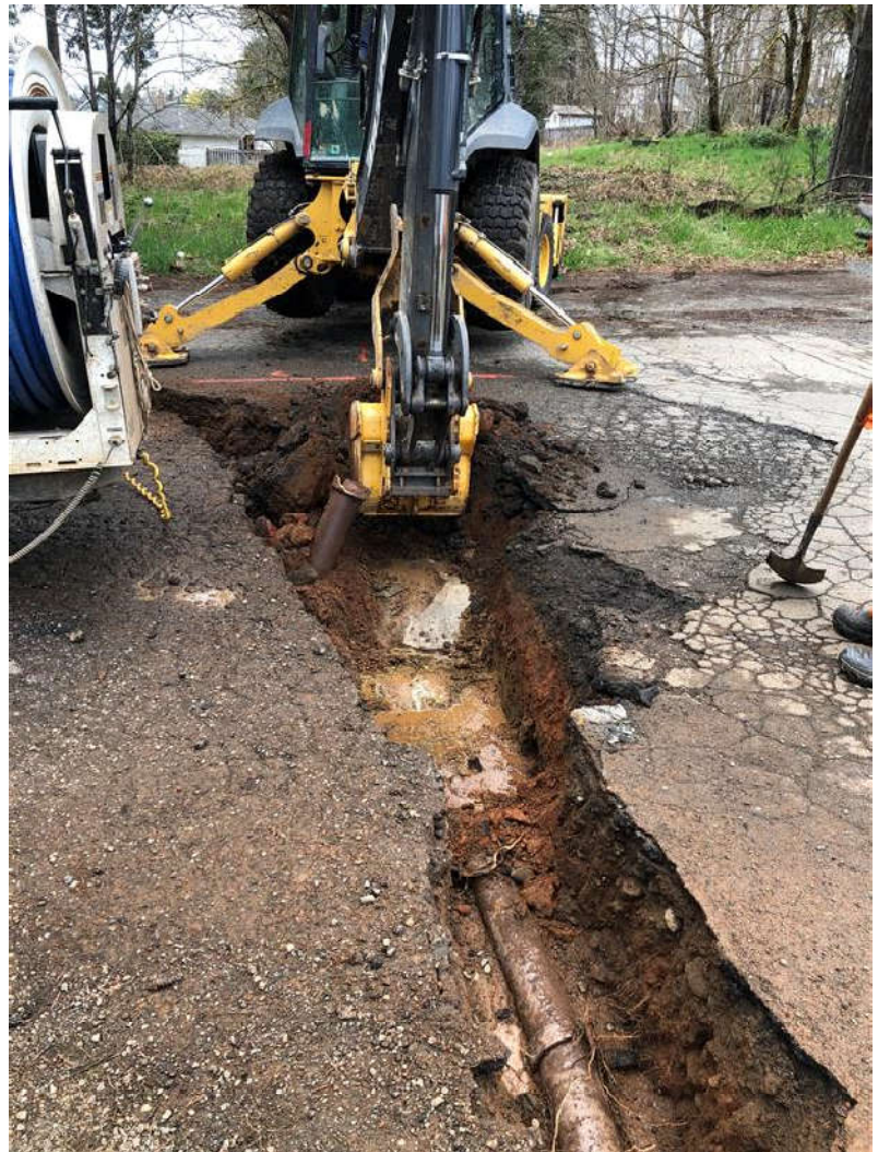
Sanitary sewer repair on Silecroft Road
