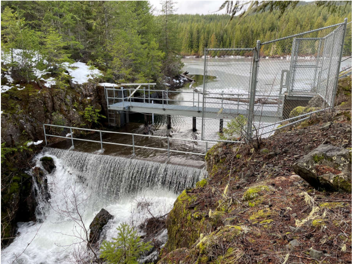
Safety fencing at Stevens Lake reservoir.
