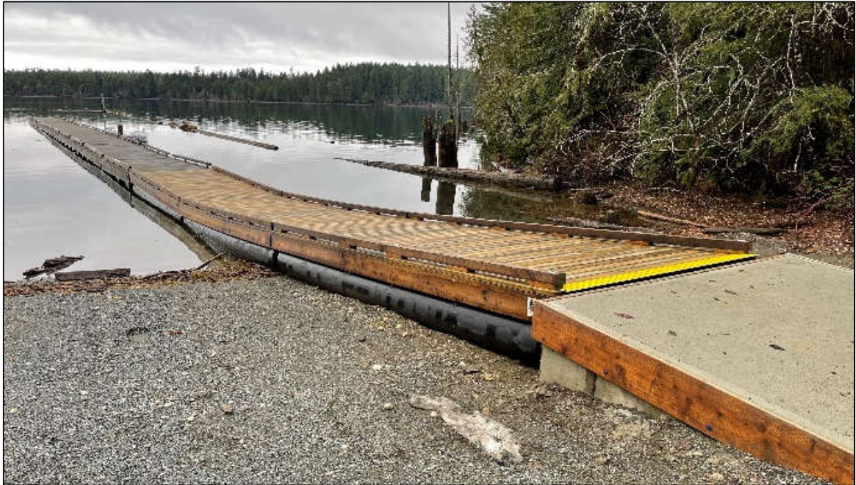
Lake Park dock replacement and realignment.
