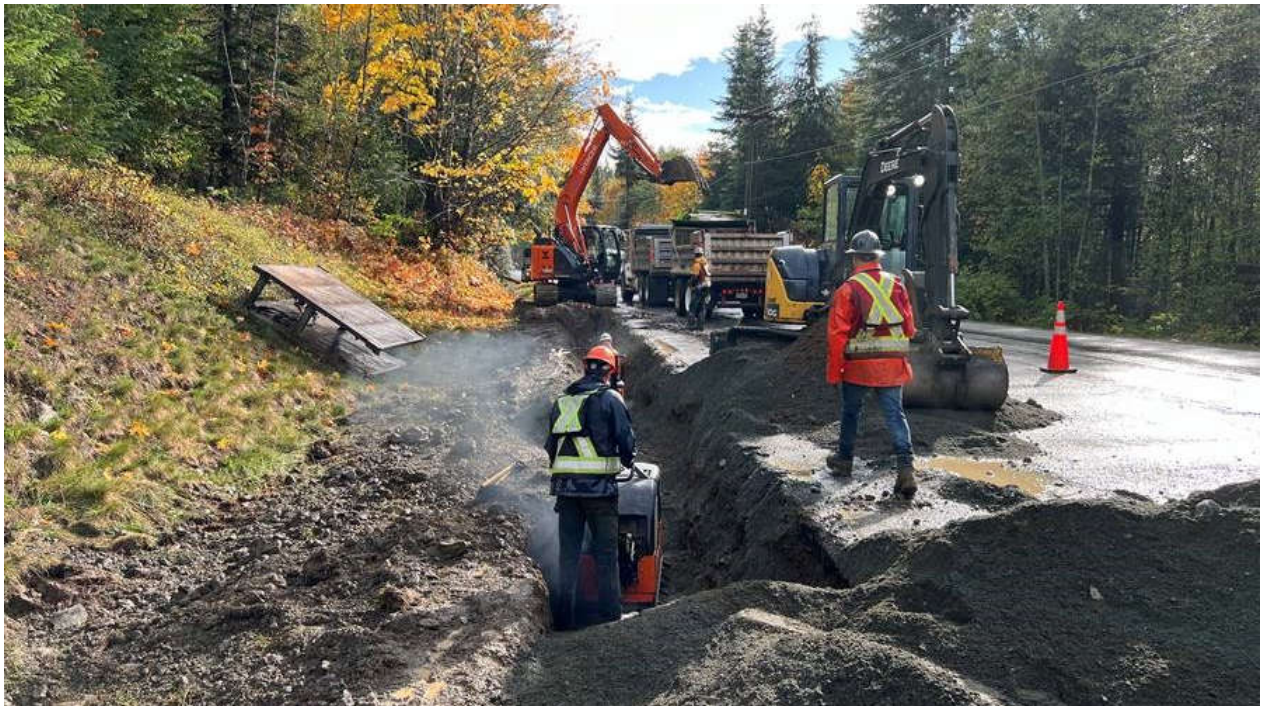
Construction of a new watermain on Union Road.
