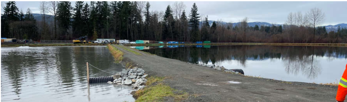
Preliminary construction work and site preparation at the wastewater treatment lagoon.
